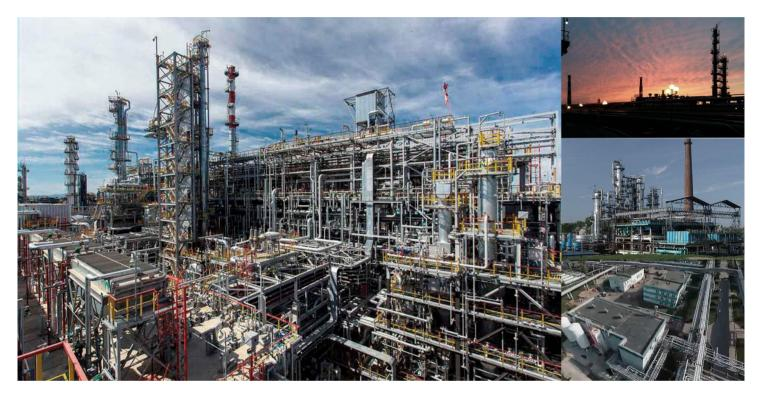
The Khabarovsk Refinery Hydroprocessing Project consisted of a major expansion of the existing Khabarovsk refinery, to increase plant capacity, improve performance and address both Russian and international requirements for the reduction of the sulphur content of kerosene and diesel products.
